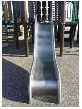
**Hazard:** The weld between the slide bedway and sidewall can crack and separate. A child's fingers can get caught in the space, posing an amputation hazard.
